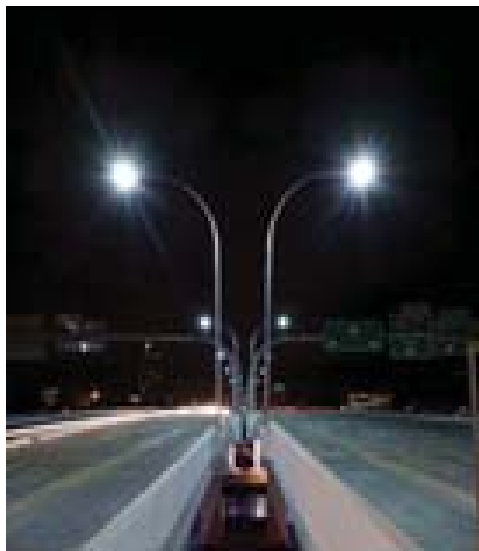
LED Lighting, I-35 Bridge, Minneapolis. (DOE)
