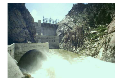
Kortes Dam & Powerplant
