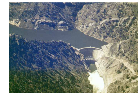
Seminole Dam (powerplant below dam)
