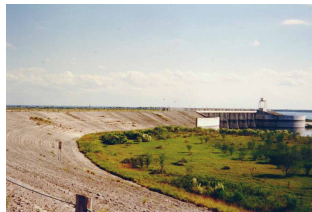
Choke Canyon (upstream face at spillway)
