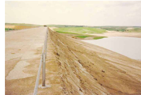
Davis Creek (upstream face)
