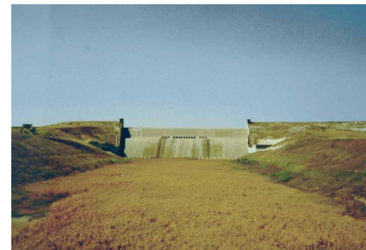
Kirwin (spillway section)
