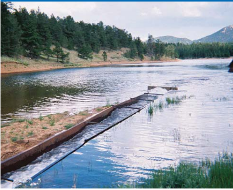
Blue River water flowing into N. Catamount Reservoir
