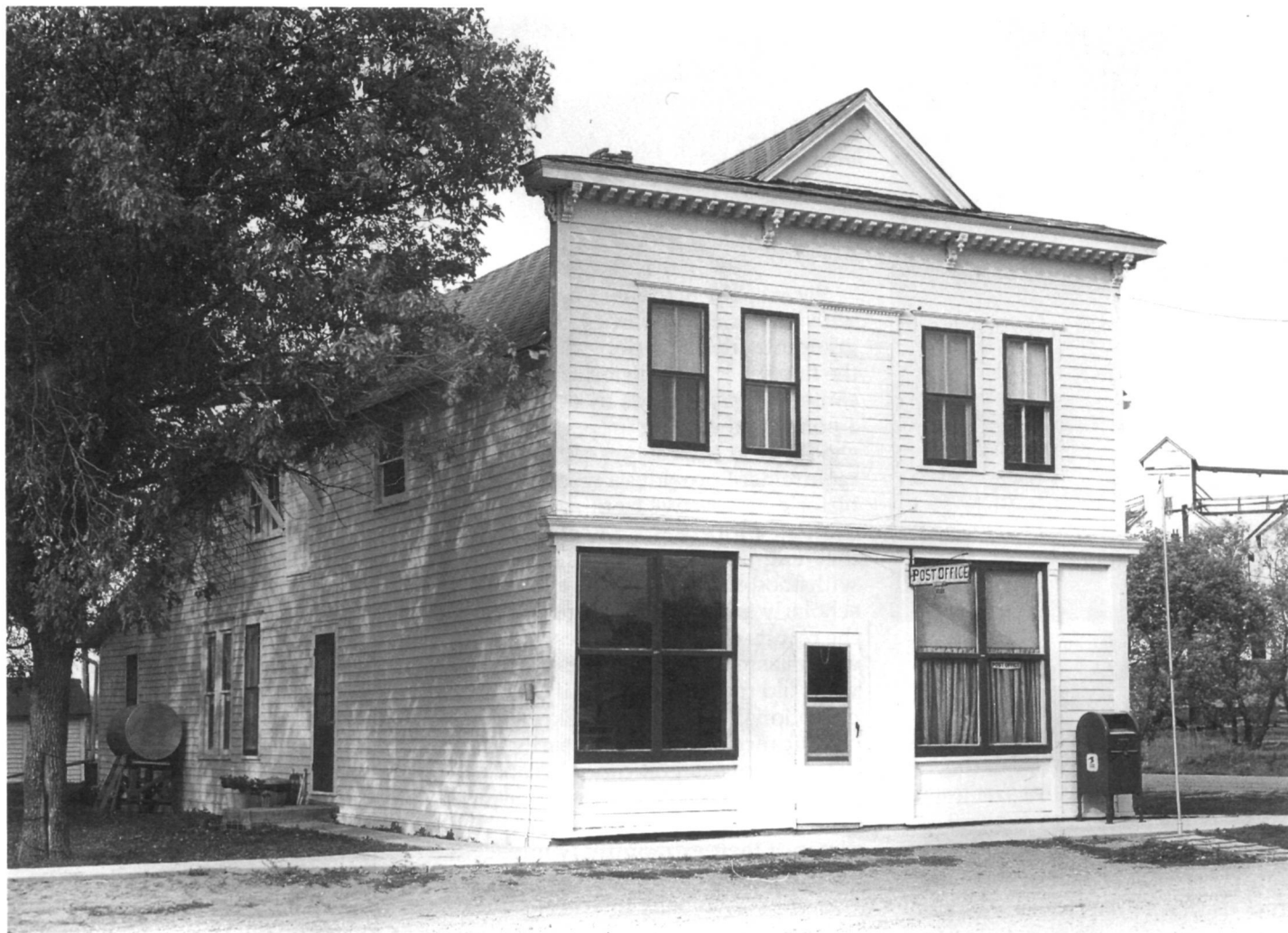
Post Office, Christine, North Dakota, ca. 1895. This building is a good example of the vernacular "Boomtown" architecture typical of North Dakota's earliest years of white settlement. Originally constructed as a residence and commercial establishment, this became a post office in 1923 after Charles Hanson, a prominent local educator, became postmaster and lived with his family in the rear portion. (State Historical Society of North Dakota)
