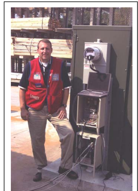
Figure 4. Carson Durham (Lowe's) Beside Simulator
