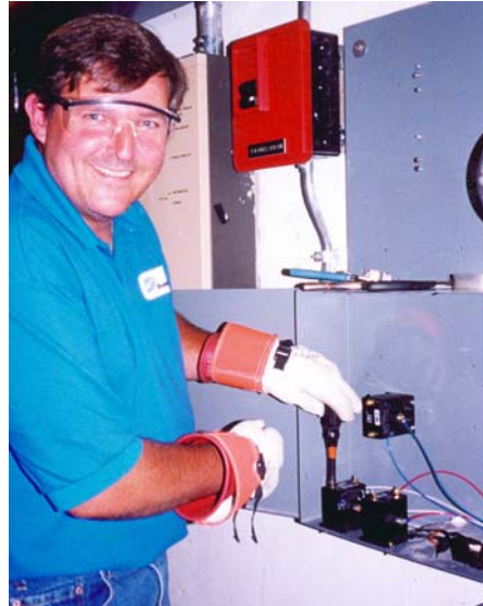
Figure 7. Jim Nystrom (Dominion) Installing CTs at CFC
