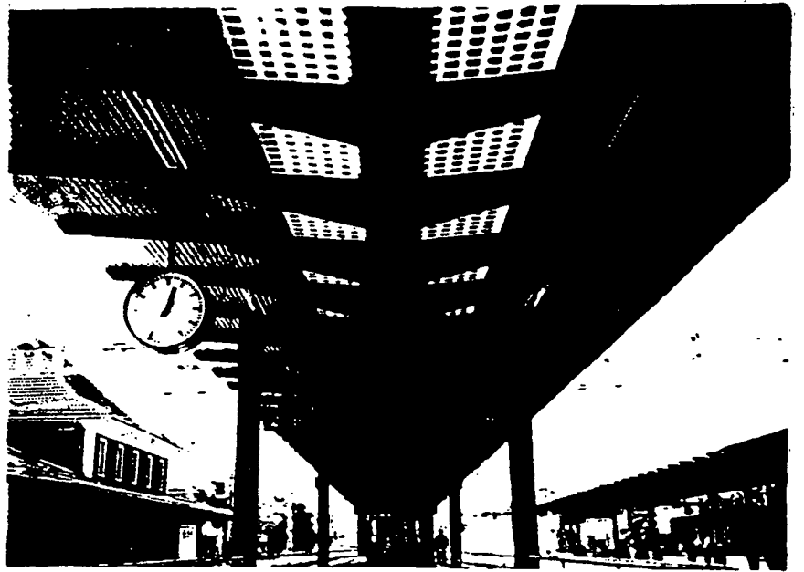
(Top: Installed from one end to the other end of the roofs)
