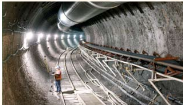
Exploratory Tunnel, Yucca Mountain.
