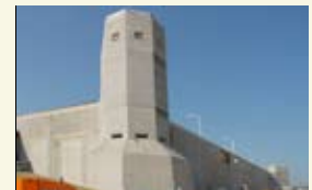
Highly Enriched Uranium Materials Facility, Y-12.
