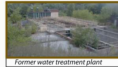
Former water treatment plant
