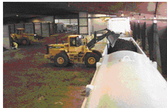
Figure 2-2: Loading Soil into Railcar at WPRAP
