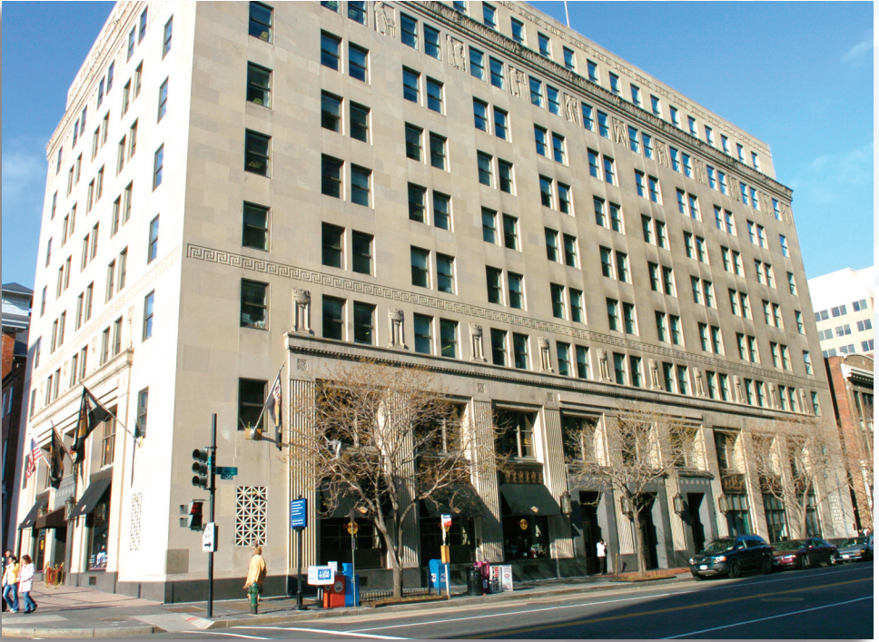
FEC Building in downtown Washington, D.C.
