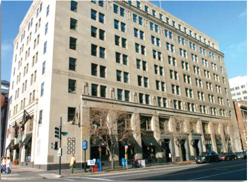
FEC Building in downtown Washington, D.C.
