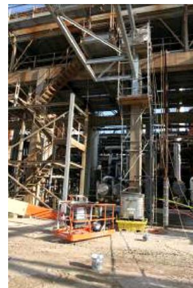
Figure 2. Another view of the work area
