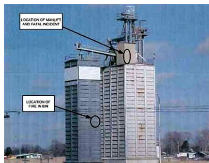
Figure 3. Location of the fire and adjoining silo
