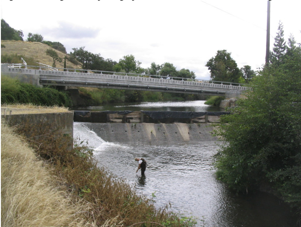
Figure 6 Tailrace downstream from Oak Street Diversion on Bear Creek August 21, 2007.
