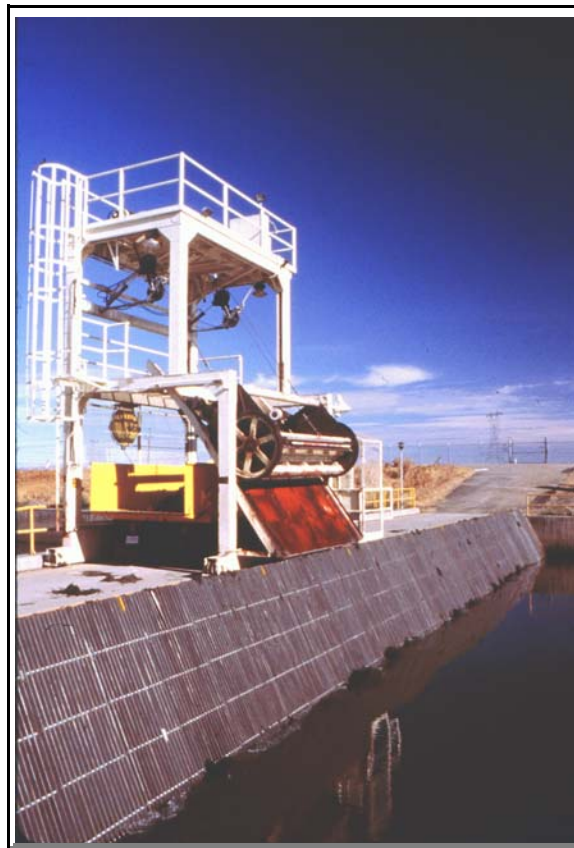
Figure 2b.—The trash rack at the intake of the TFCF. This structure is cleaned regularly by TFCF crews. The Datasonde was installed behind this structure.
