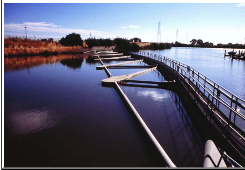
Figure 2a.—Looking eastward at the Old River from the TFCF intake. The debris and trash boom is located at the inlet of the TFCF.
