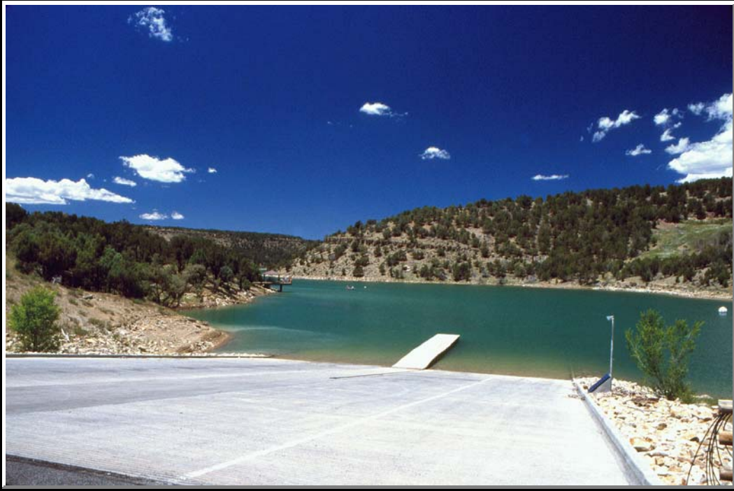
Figure 4a.—The main boat launching ramp at Ridgway Reservoir, looking north.
