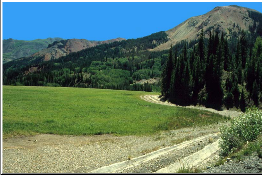
Figure 5c.—A tailings deposit remediation project north of the Idarado Mine. The materials have been covered, revegetated, and a drainage system has been installed (lined channels in the foreground).
