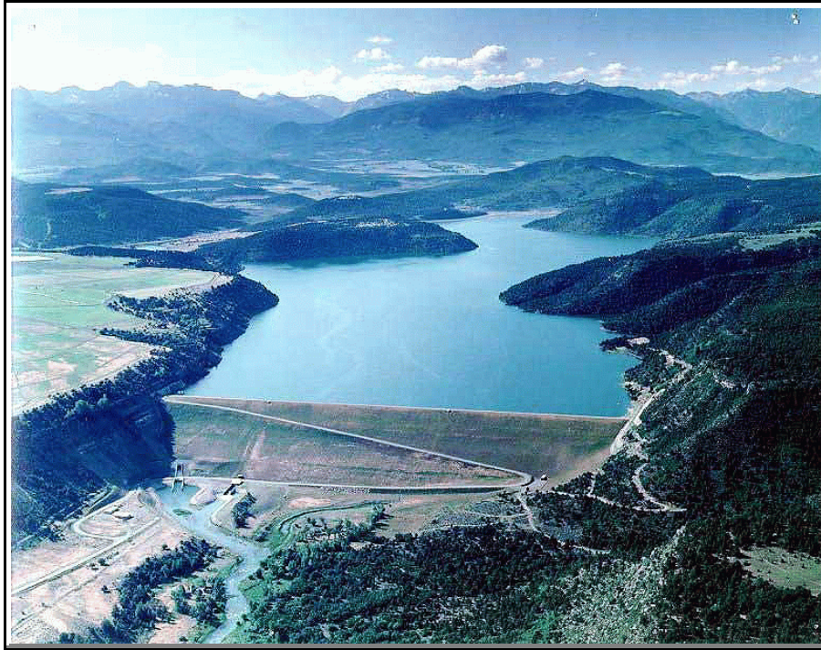
Figure 1.—Aerial view looking south at Ridgway Dam and reservoir (Bureau of Reclamation, 2000).
