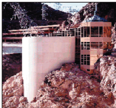
Hoover Dam Visitor Center.
