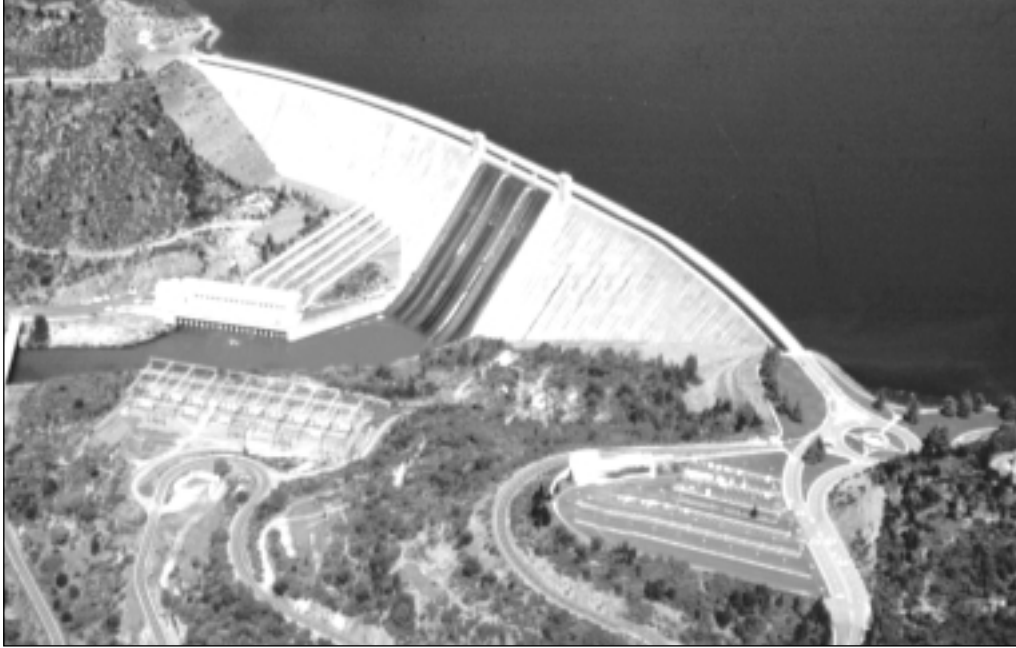
Bureau hydroelectric facilities like this one at Shasta Dam helped to mitigate the energy shortages plaguing many areas of the West.
