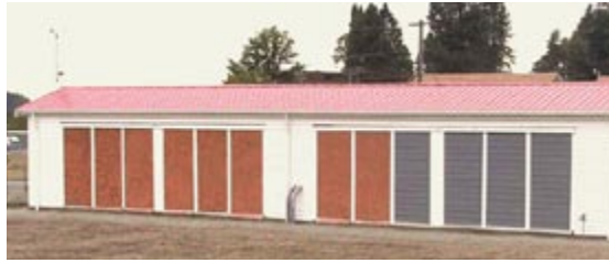
Washington State University is using the Natural Exposure Test Facility (NET), established in 2003 to evaluate the effects of heat, moisture, and ventilation on wall assemblies.
