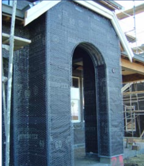
Housewrap provides a drainage plain behind stucco and other finishes.
