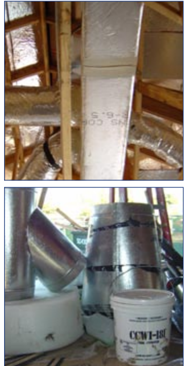
Mastic provides the most reliable duct sealing method for new construction.
