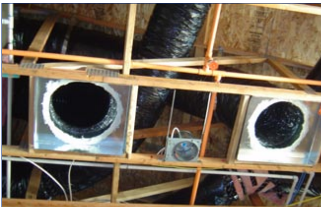
Careful duct sealing with mastic helps improve comfort and energy efficiency at low cost.
