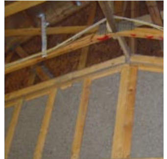
Blown-in wall insulation
