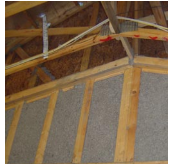
Blown-in wall insulation
