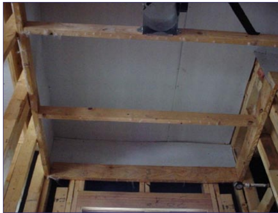
Draftstopping applied at the top of the second floor bulkhead.
