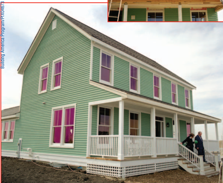
High efficiency, argon-filled windows with low-emissivity glass were installed on this Building America home in the Prairie Crossing community in Grayslake, Illinois. Prairie Holdings Corporation was the builder partner (BSC).
