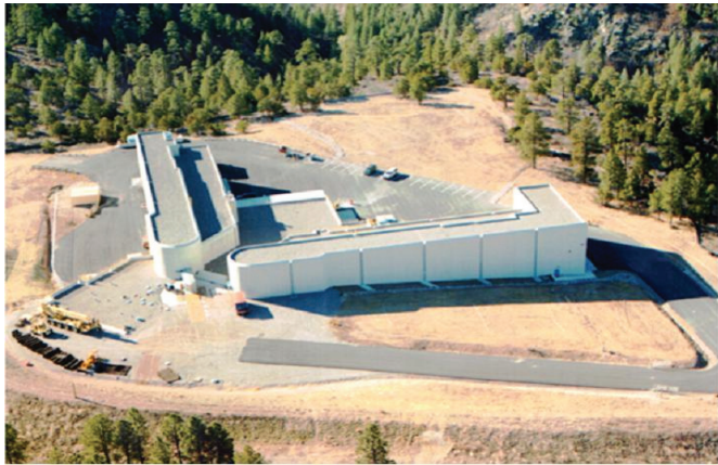
DARHT: Aerial view of the the Dual Axis Radiographic Hydrodynamic Test facility at Los Alamos.
