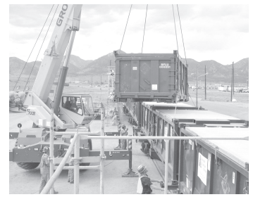
First rail shipment at Rocky Flats.
