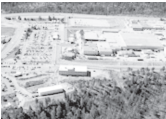
Las Alamos National Laboratory Plutonium Facility.
