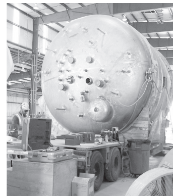
The pipefitter is working on the nozzle for the High-Level Waste Facility located at the Office of River Protection.
