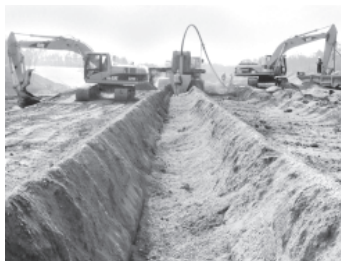
Hydrologic isolation activities for Solid Waste Storage. This includes employing a state-of-the-art trenching technology that ensures that the project meets the regulatory requirements for reducing groundwater infiltration into the Waste Burial Grounds at Y-12.
