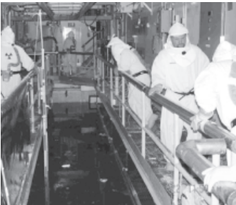
Team members of the K Basins Decontamination and Decommissioning project begin pouring grout to permanently fill and secure the discharge chute.
