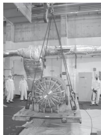
Filling and transporting a Cask from L-Area to the E-Area burial ground, for final disposal at Paducah.
