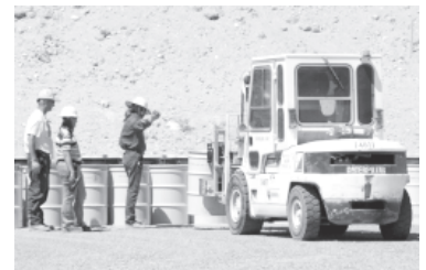
Disposal Operations Personnel Guide a Forklift to Position a Drum Containing Low-Level Waste Within the Pit 9 Grid System at the Area 5 Radioactive Waste Management Site located at the Nevada Test Site.
