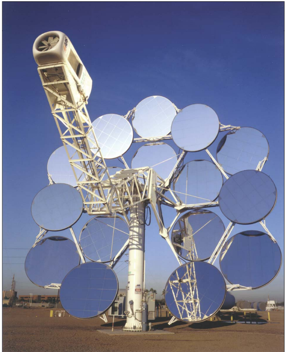
Dish Stirling Solar Power System at the Arizona Public Service Solar Test and Research Center.
