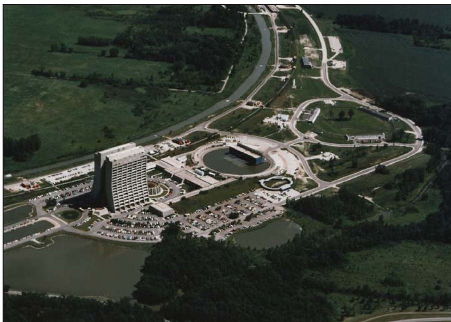
Aerial photograph of Fermi National Accelerator Laboratory, Batavia, Illinois.
