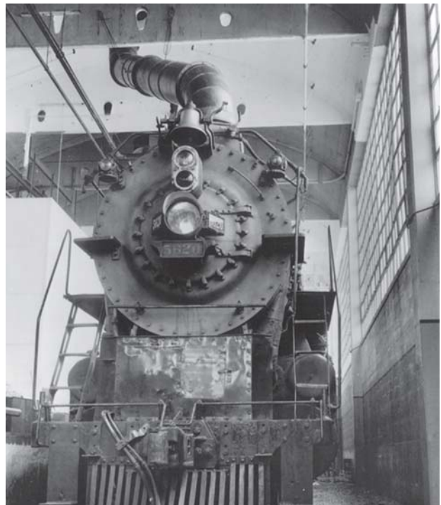
AN UNUSUAL SOLUTION: In the early days, the facility experienced a shortage of steam to produce plant heating. Two locomotives were driven onsite and hooked up to plant steam lines.
