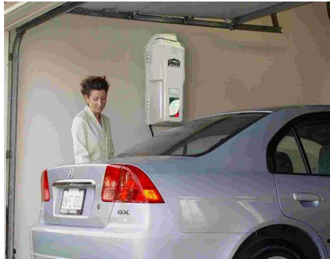
Figure 6: “Phill” Home Refueling Appliance (courtesy of American Honda and FuelMaker)
