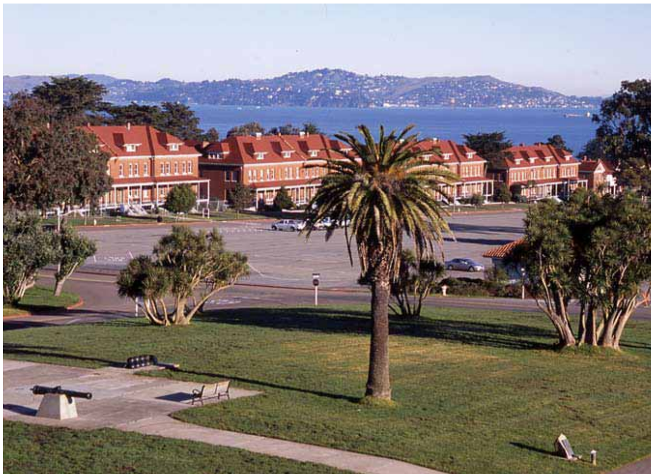
View north of the Montgomery Street Barracks
