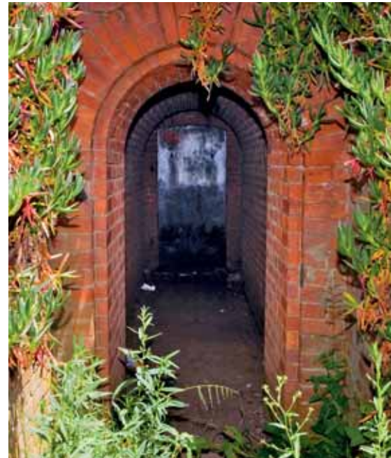
Entrance to a magazine at Battery East built in the 1870s.
