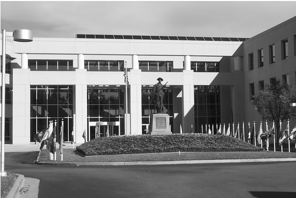
The Army National Guard Readiness Center in Arlington, Virginia. (National Guard Bureau)
