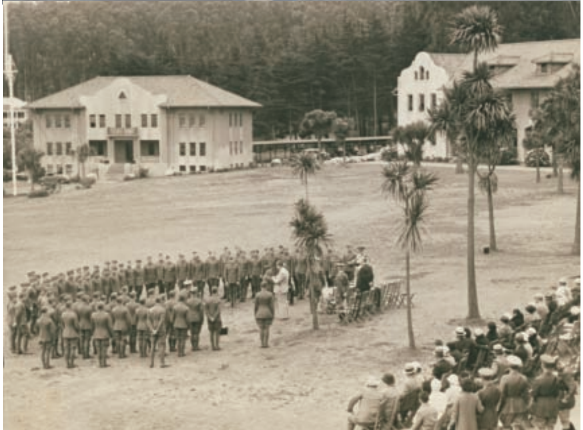
Top: Presidio Trust project manager Peter Foley and architectural conservator Christina Wallace at Fort Scott. Bottom: Fort Scott in the 1930s.
