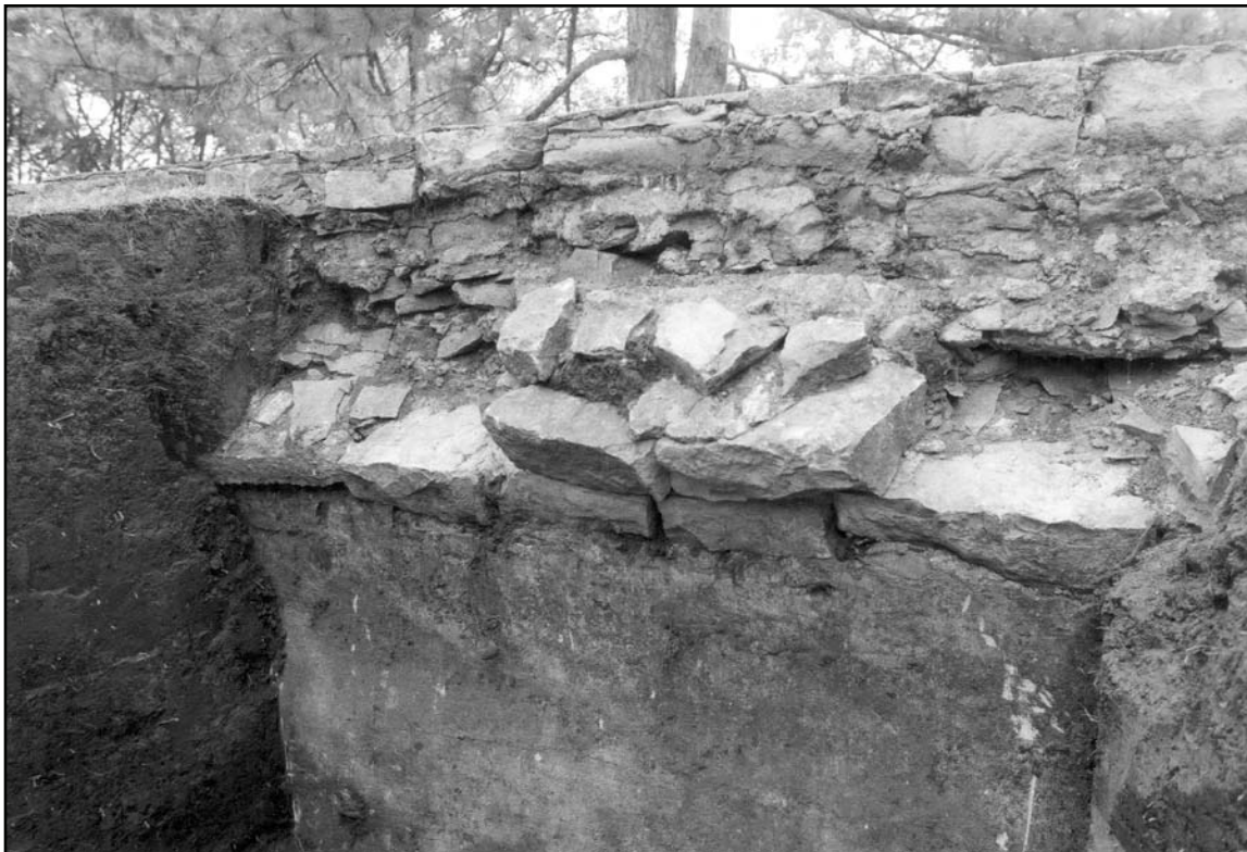
Figure 9. East wall of the cistern showing the spring line of the roof vault, which is tied into the inner face of the retaining wall.
