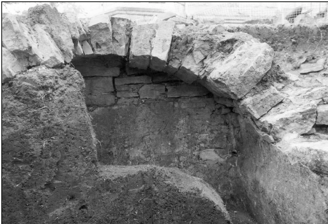
Figure 12. Close-up of the south interior cistern wall. The probable iron inlet pipe is visible at the lower right.
