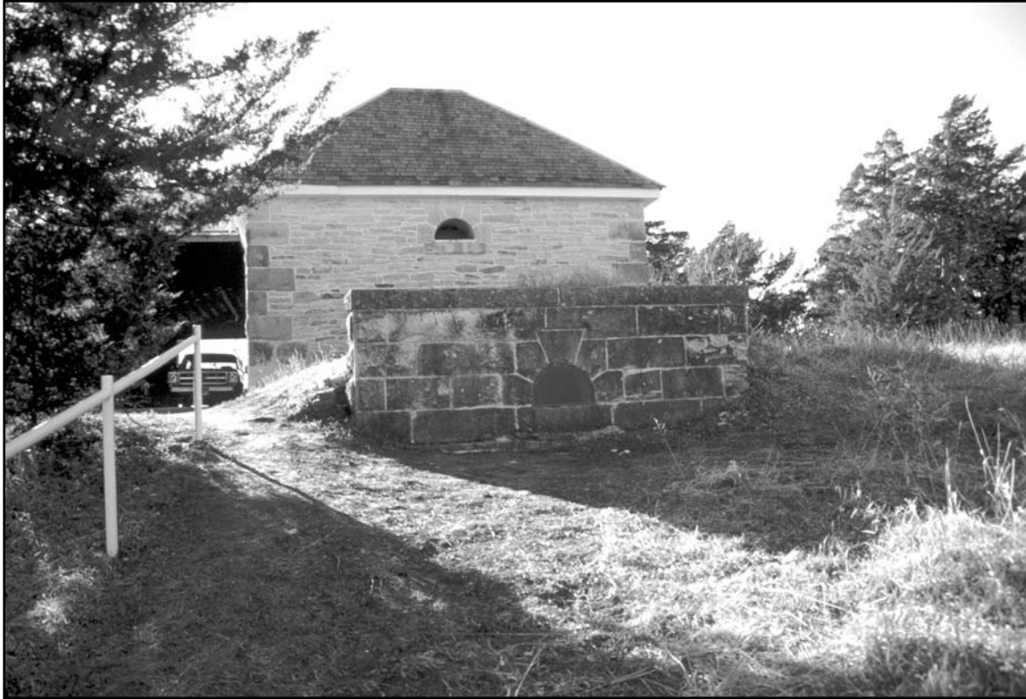
Figure 3. Cistern below the east side of the ice house, Spring Hill Ranch Headquarters complex. View to west from behind the main ranch house.
