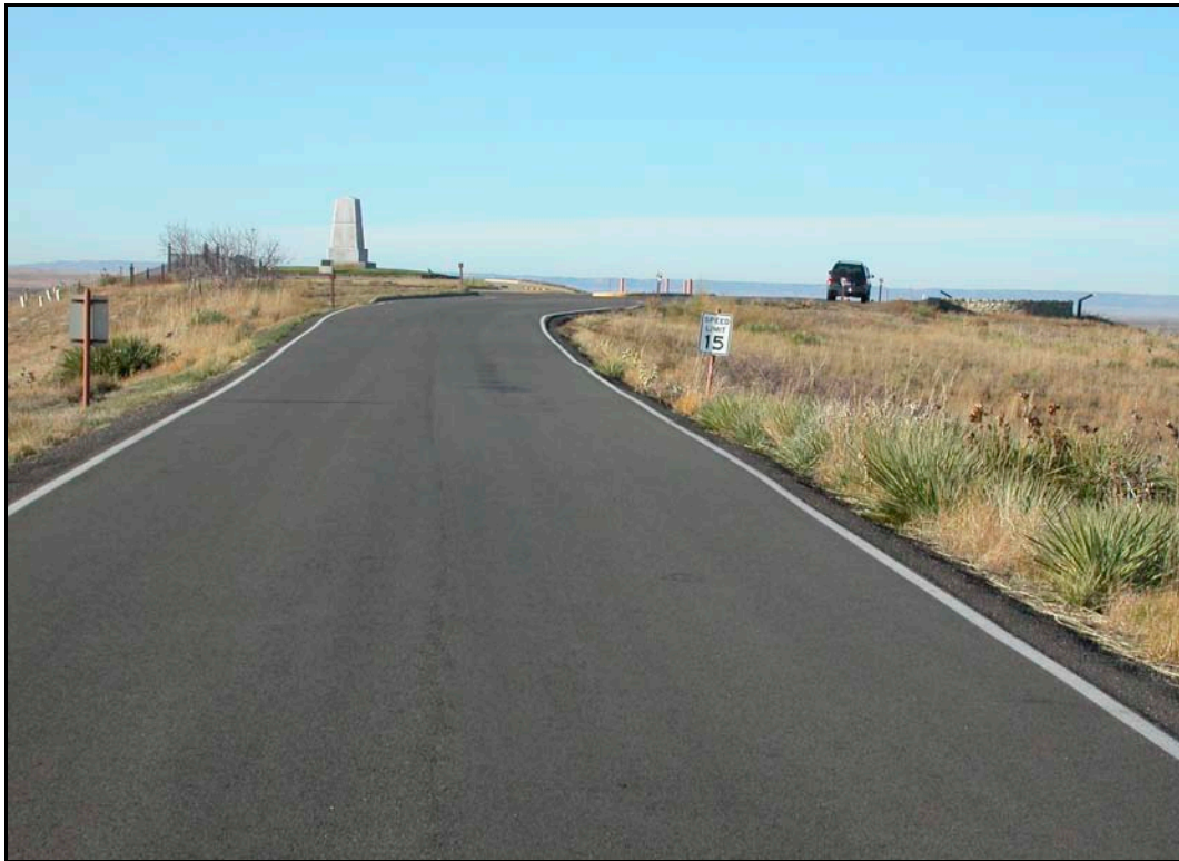
Figure 5. A 2004 image of the same area as Figure 4 showing the road alignment.
