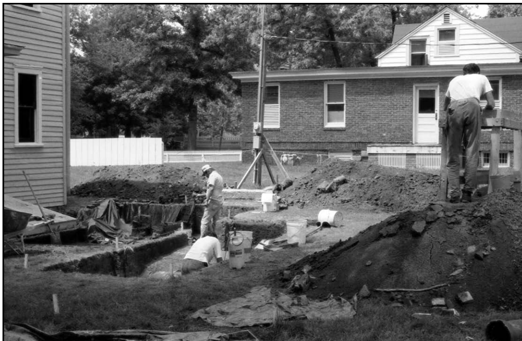
Figure 7. Overview of block excavation area.
