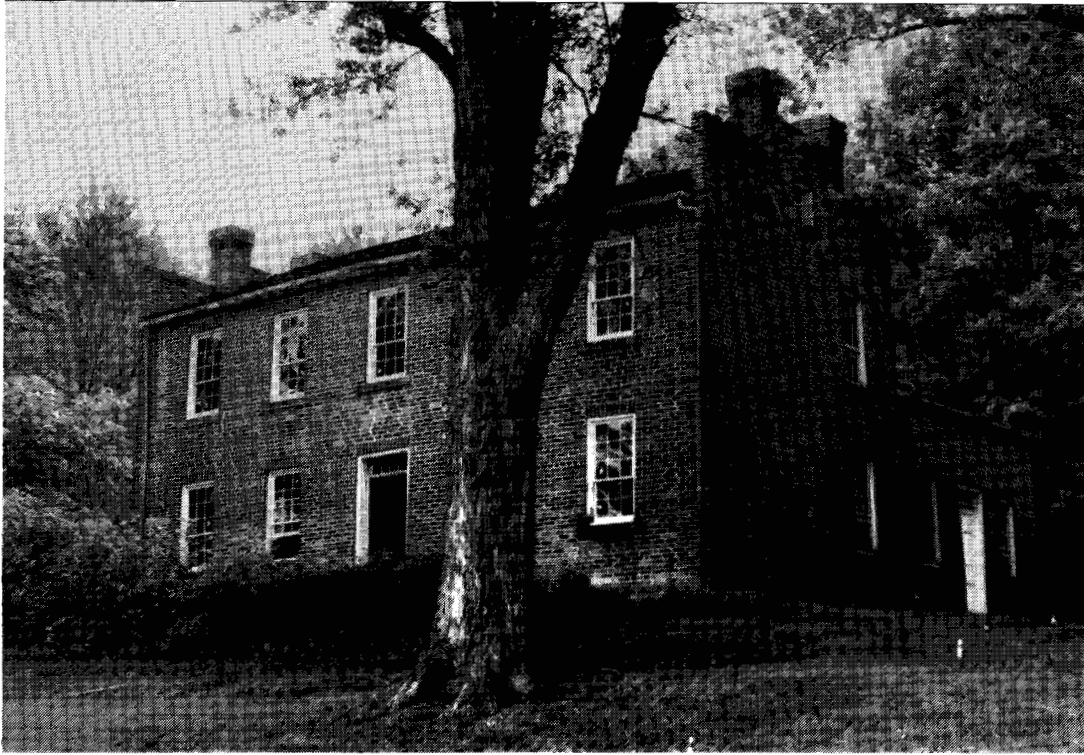
Figure 6. West and south elevations of the Frazee-Hynton House.
