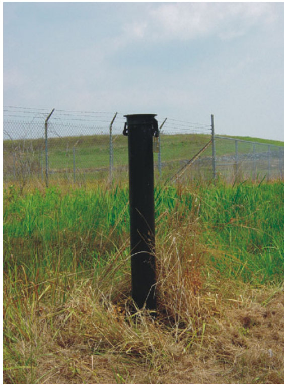
Perimeter Gas Monitoring Probe
