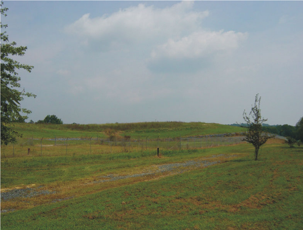
View of the Bush Valley Landfill
