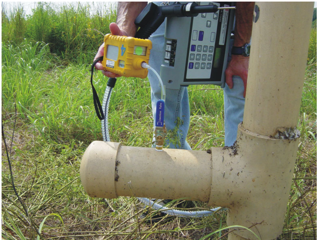
Landfill Gas Screening at a Passive Vent
