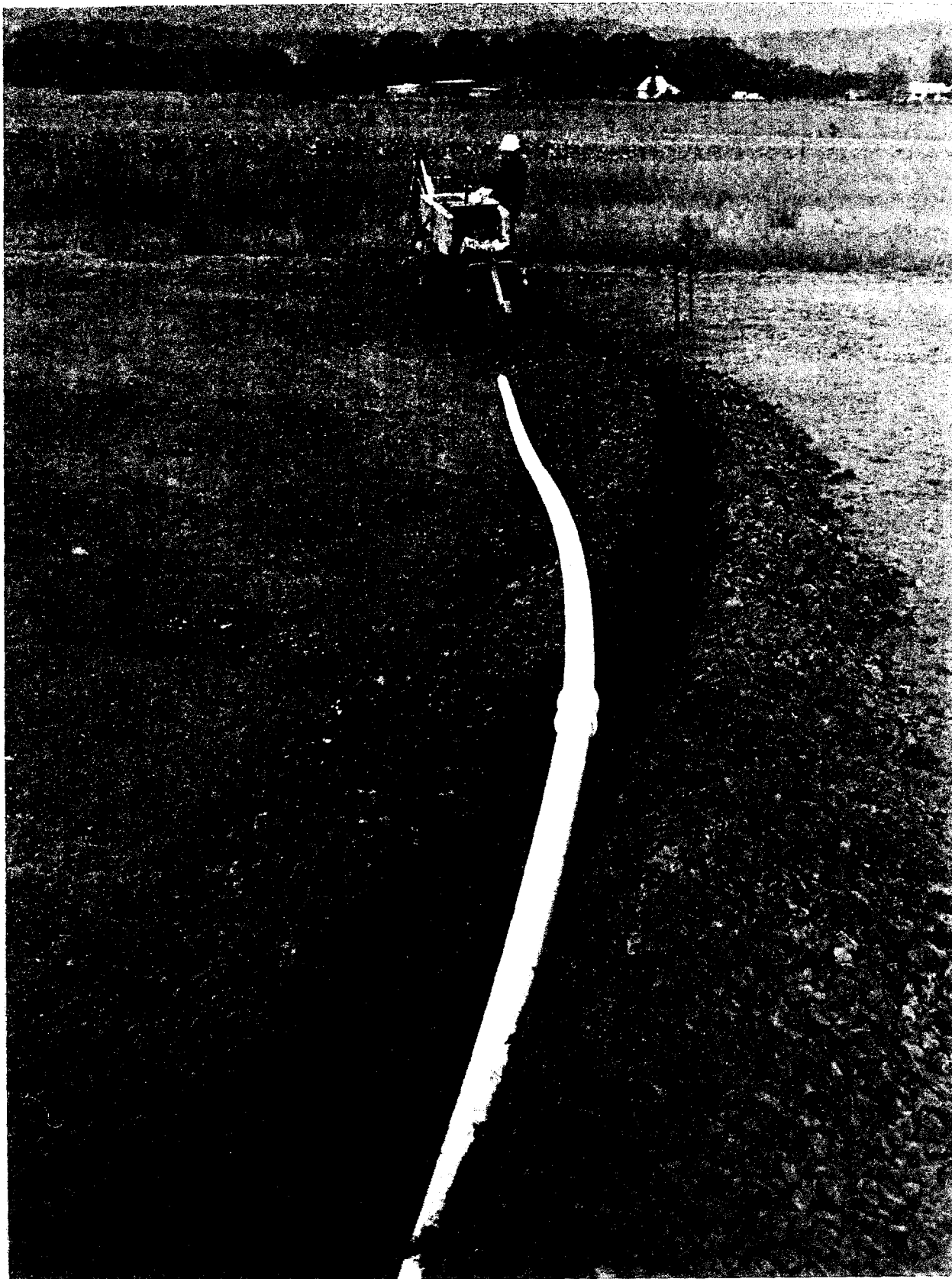
Figure 1-1. Installation of pressure sewer main.
