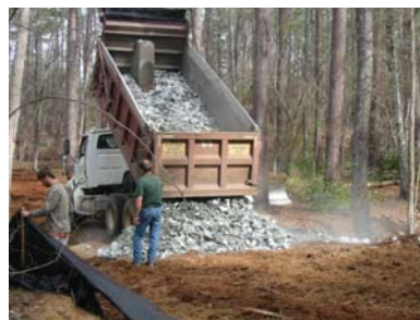
Figure 3 - Road construction introduces off-site materials which may contain invasives.
