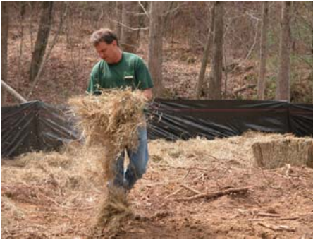
Figure 19 - Applying mulch for soil stabilization
