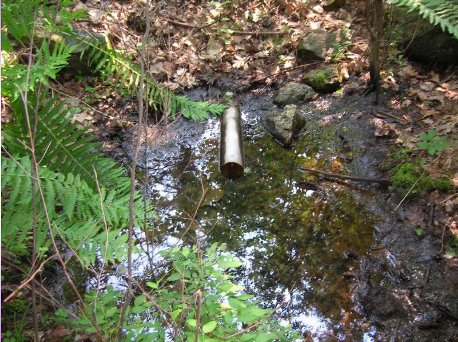
Discharge to Ground - Pelham, NH
