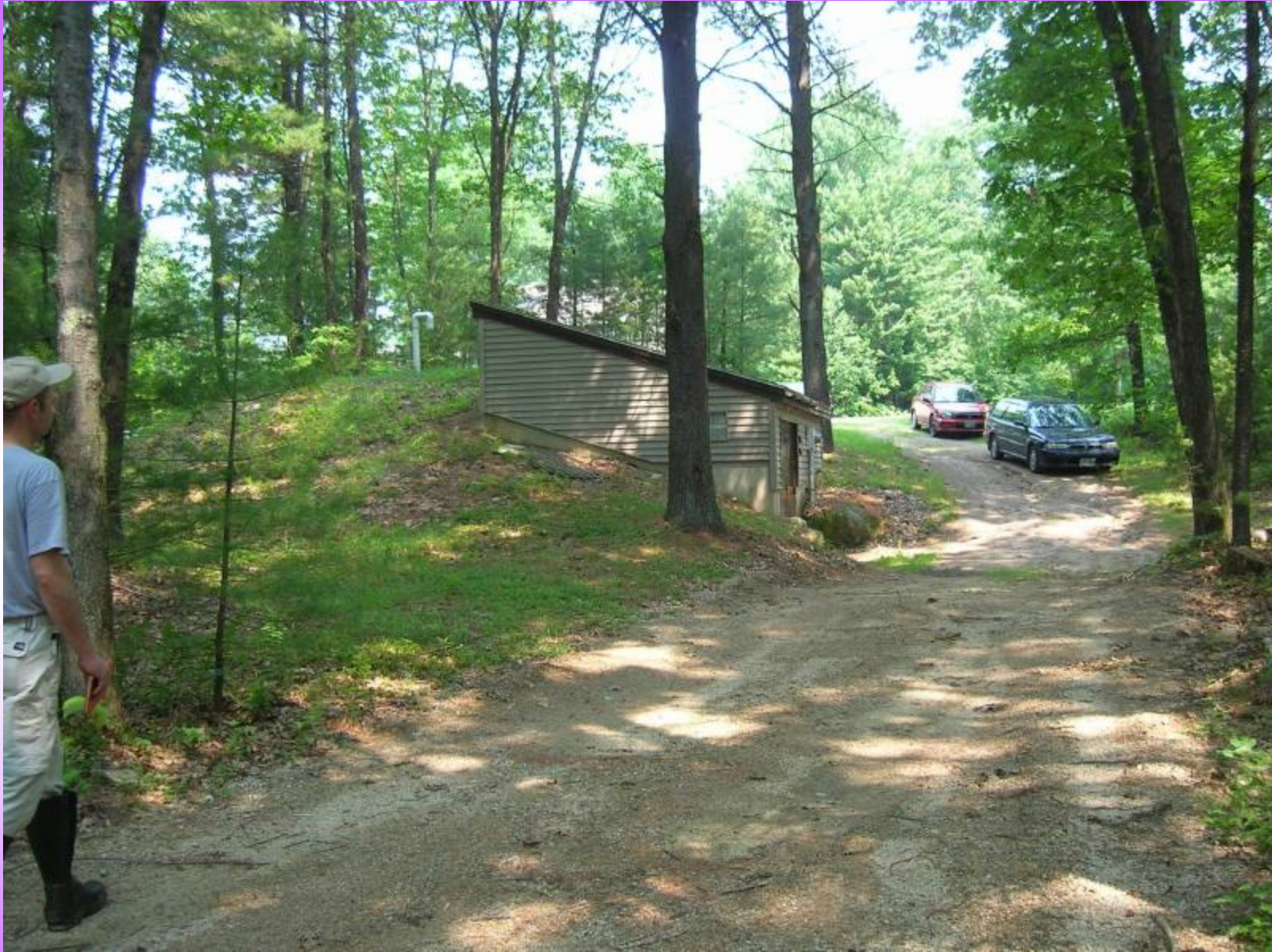
Well House and Treatment - Bedford, NH
