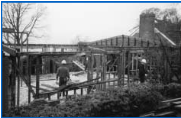
Deconstruction of a single-family home in Portland, Oregon.
