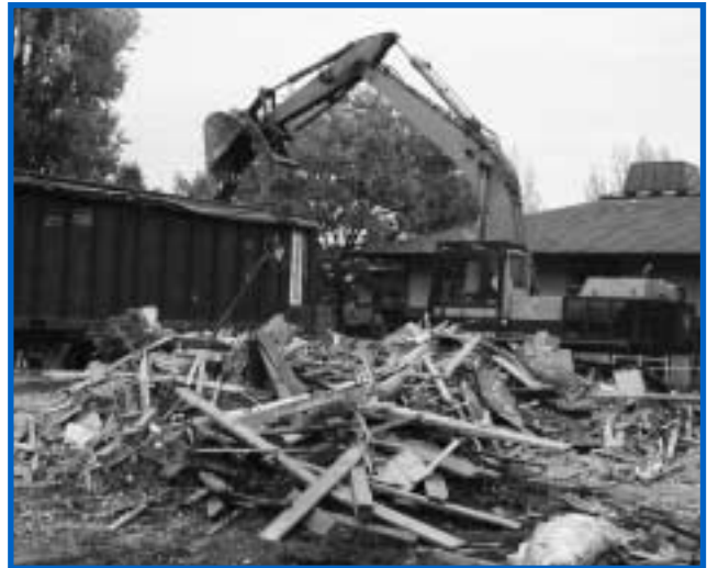
The demolition of wood-framed buildings results in the wood members being broken up, intermixed with other materials, and greatly reduced in value.
