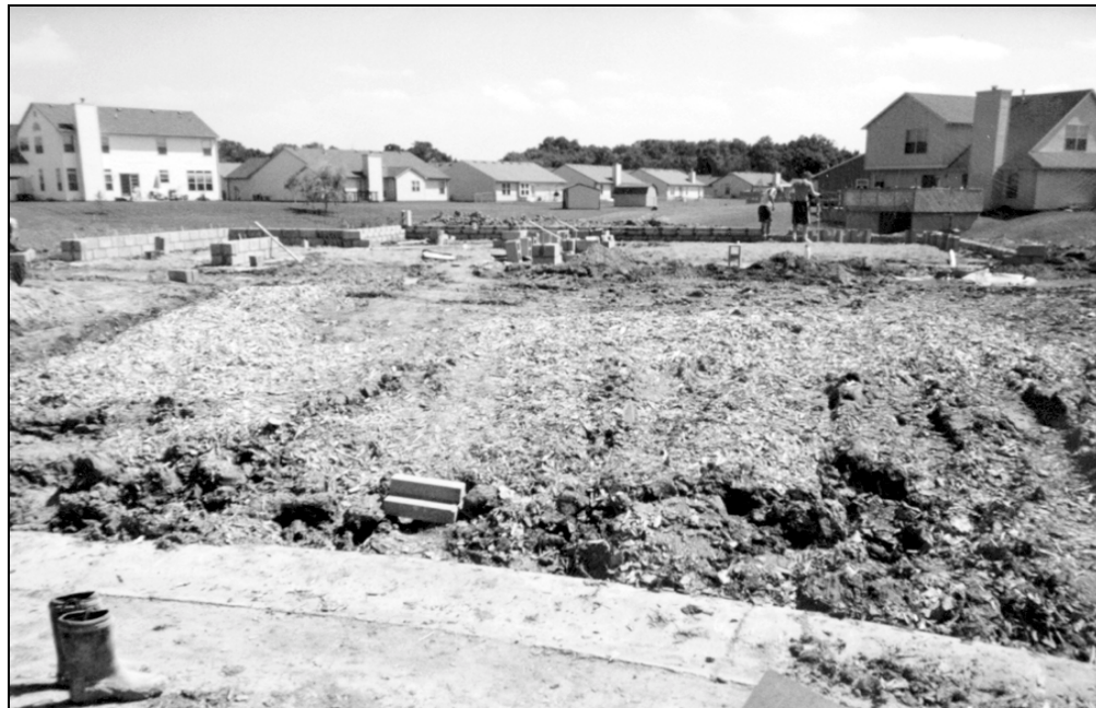
Photo 5 – Site with processed material used for erosion control
