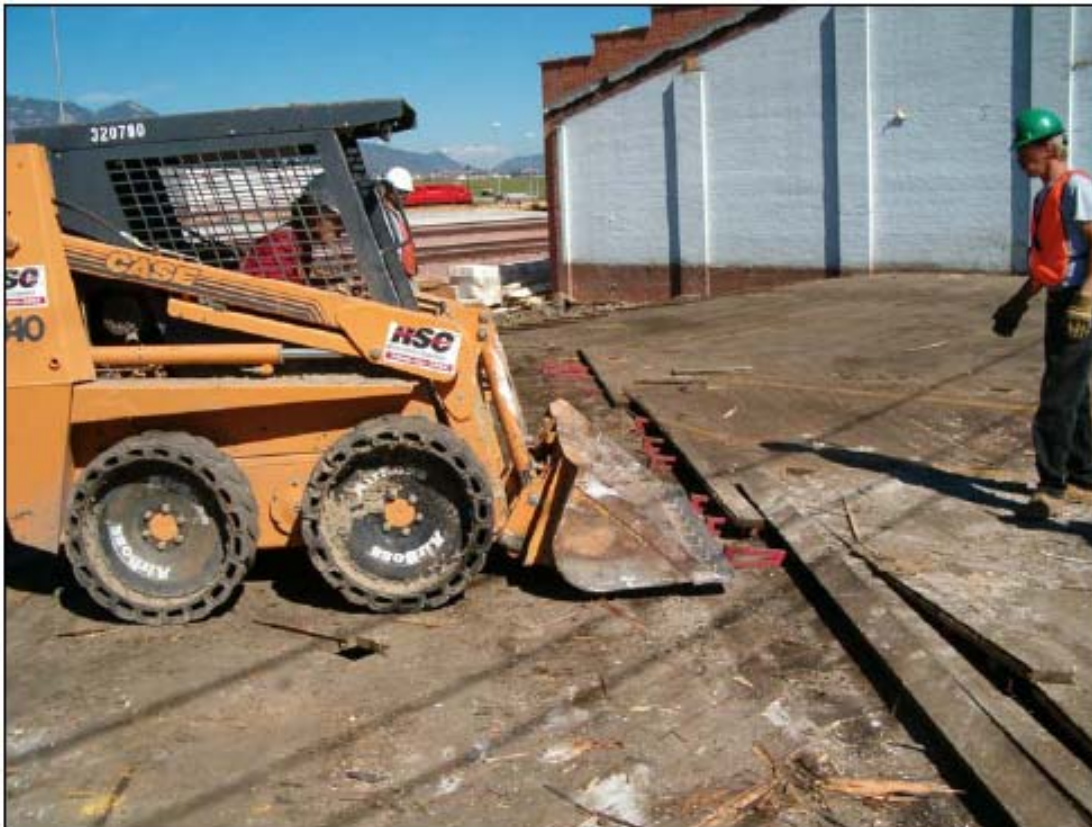
Figure A16. Removing flooring with skid-steer.
