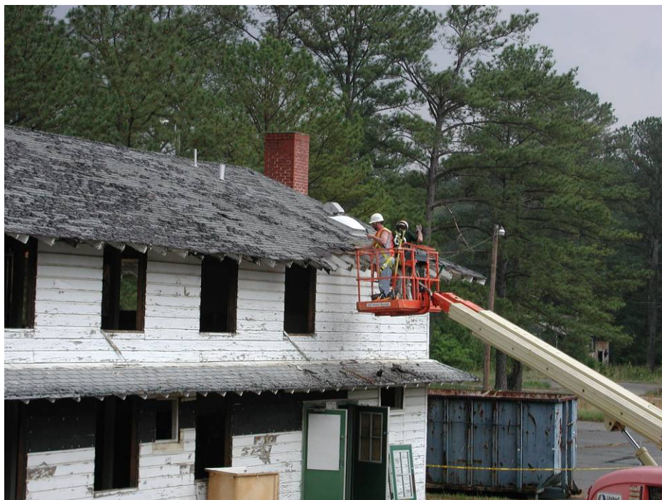
Figure A3. Removing eaves at Fort McClellan.
