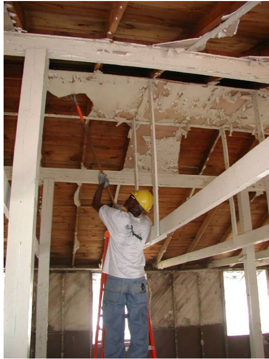
Figure A2. Removing drywall at Fort McClellan.
