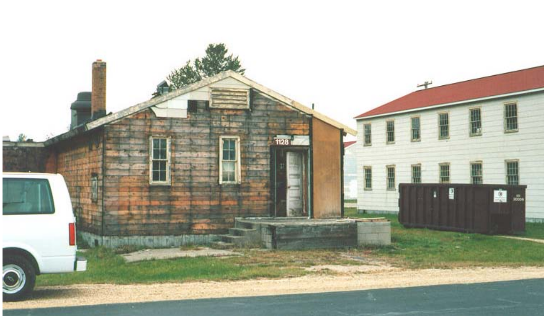
Figure A21. WWII building at Fort McCoy.
