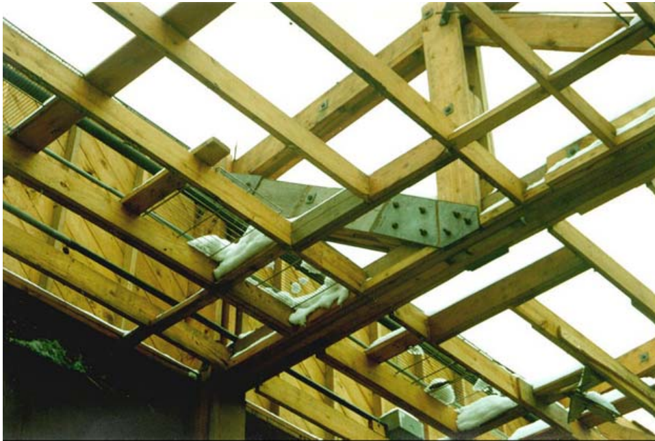
Figure A23. Roof trusses of WWII-era theater.
