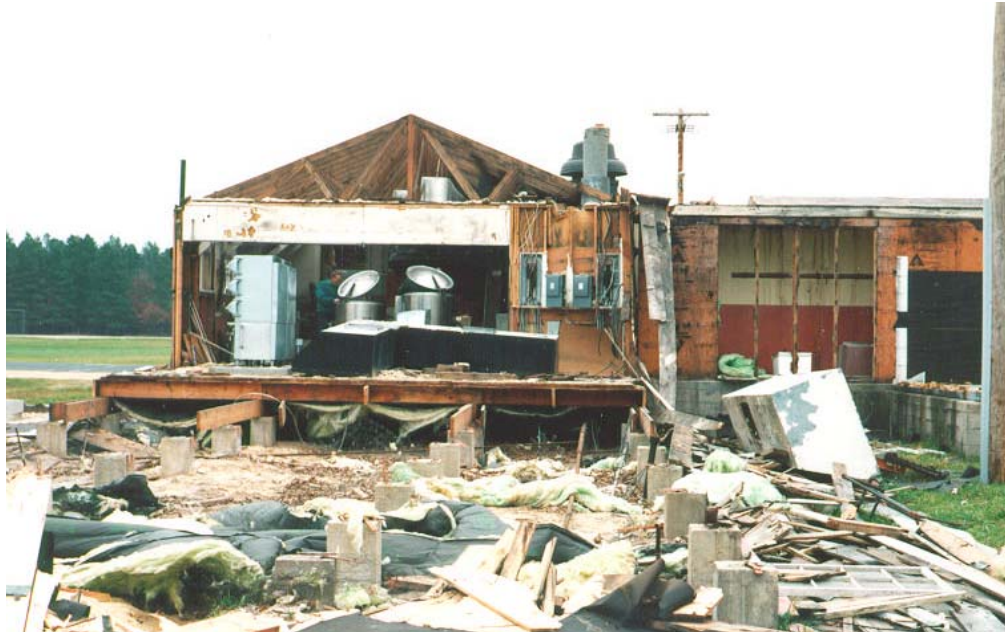
Figure A22. Fort McCoy mess hall under deconstruction.
