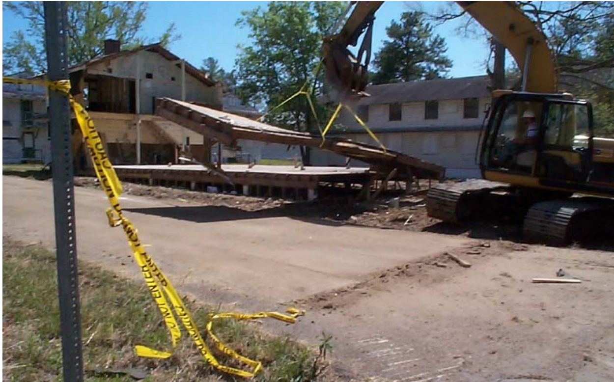
Figure A5. Floor panelization at Fort McClellan.
