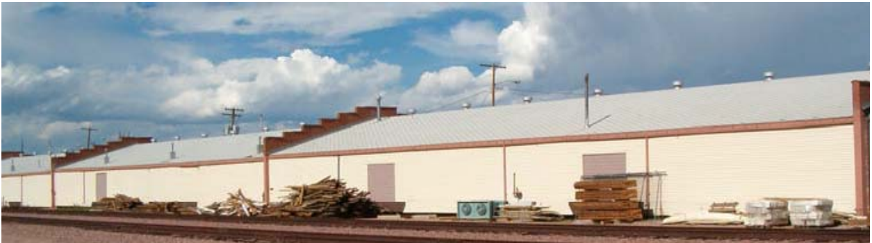
Figure A11. Building 227 at Fort Carson.
