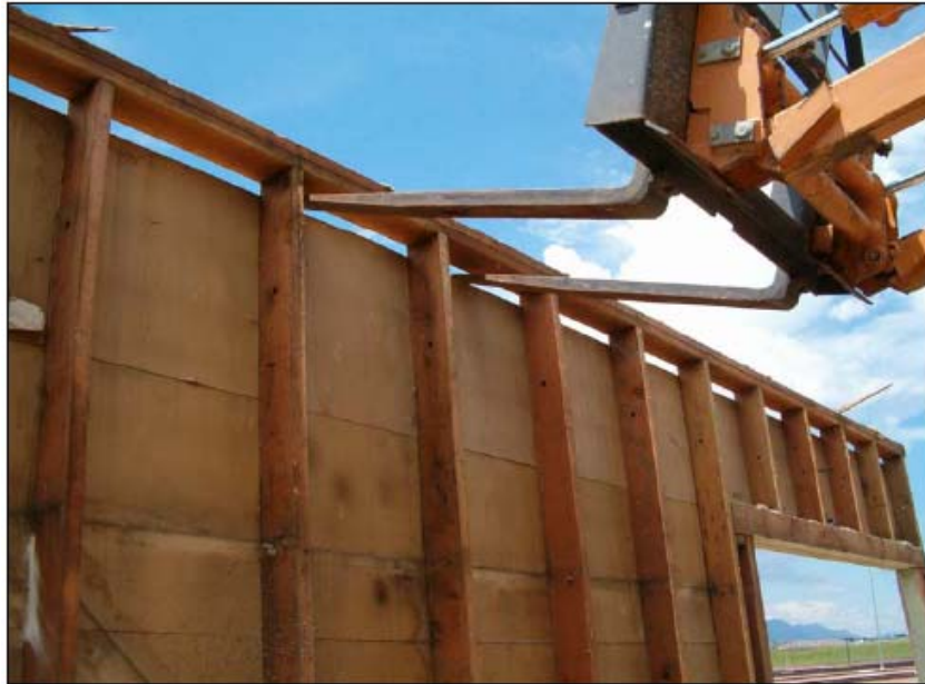
Figure A15. Reach forklift removing exterior walls
