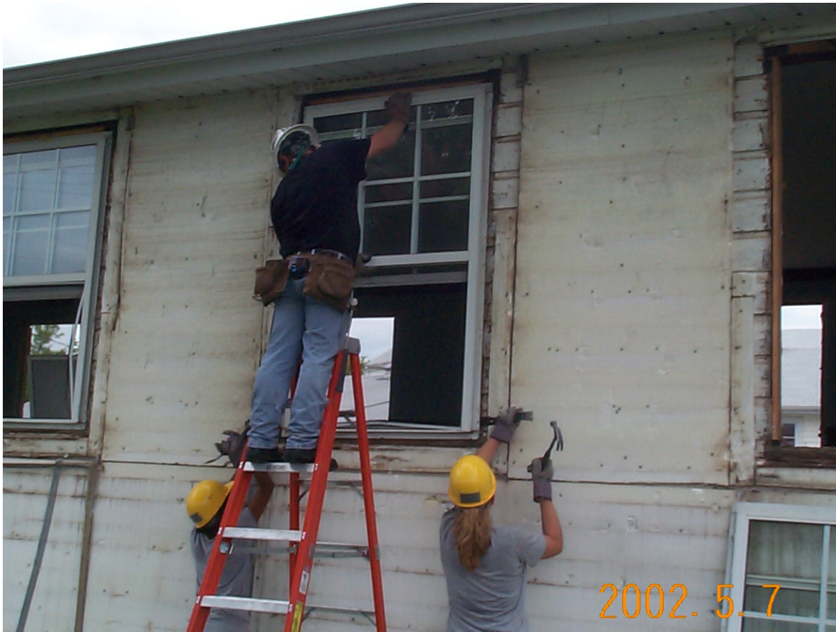
Figure A4. Removing windows at Fort Campbell.
