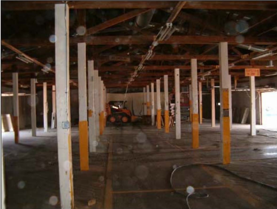
Figure A14. Interior view of columns and roof structure in building 227.
