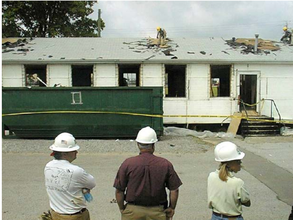
Figure A7. Building deconstruction at Fort Campbell.
