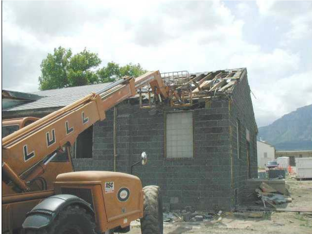
Figure 12. Reach forklift removing a roof section.
