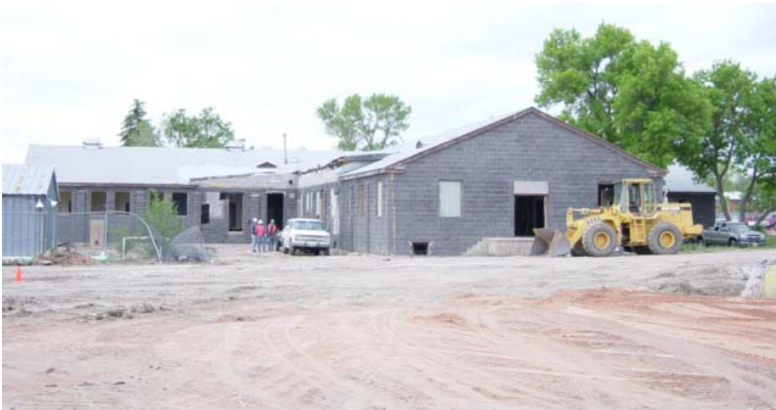
Figure A10. Building 6286 at Fort Carson, shortly before deconstruction.
