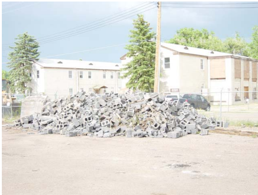
Figure A18. Cinder block intended for recycling.
