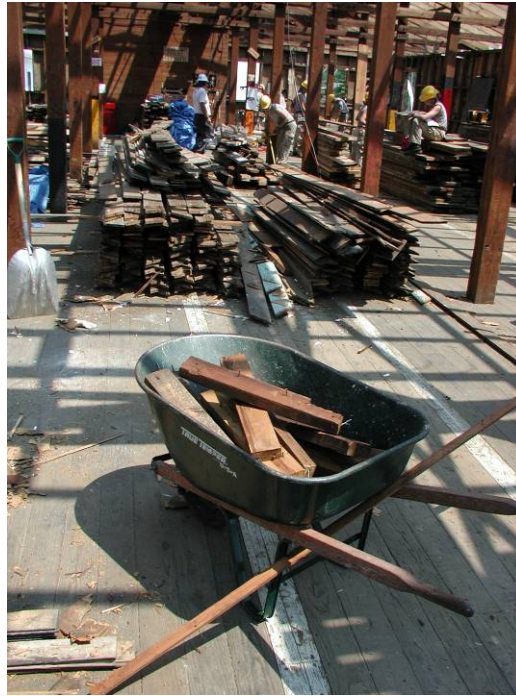
Figure A9. Stacking salvaged wood at Fort Campbell.
