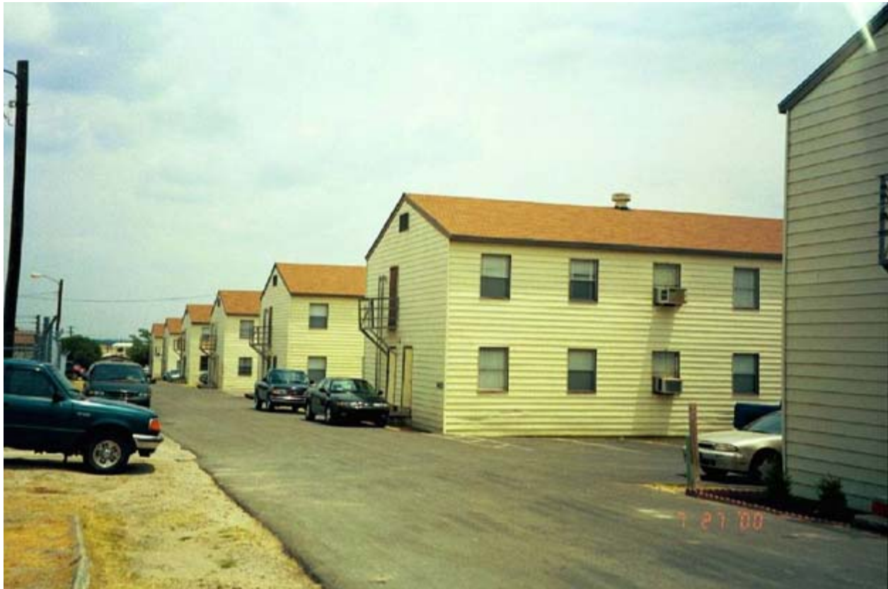
Figure A1. Typical WWII-era, wood-frame buildings at Fort Hood.
