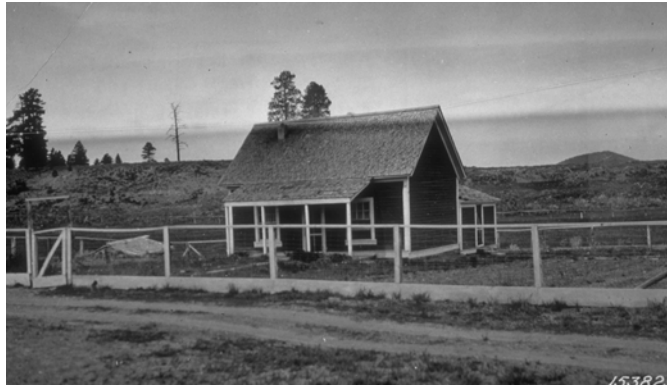
Daves Hollow Guard Station, 1921
