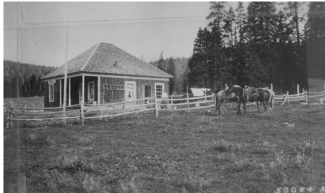
Little Valley Ranger Station
