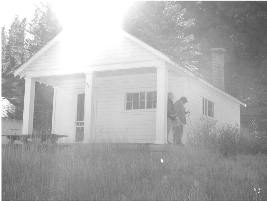
Photo: Cowpuncher Guard Station Dwelling
