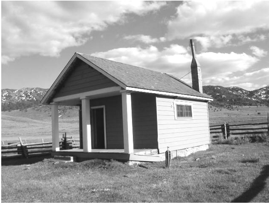
Photo: Bear Valley Guard Station Dwelling
