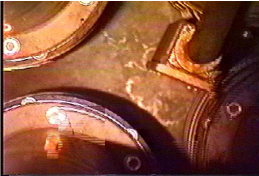
Typical of Boric Acid Staining on Cooling Shroud as Found from 2R15 Inspections
