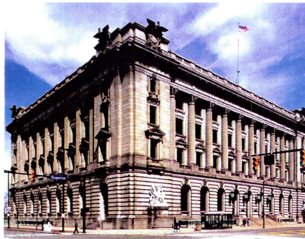
Arnold W. Brunner's U.S. Post Office, Custom House, and Court House, an early-20th-century landmark in downtown Cleveland, has undergone a $45 million restoration.
