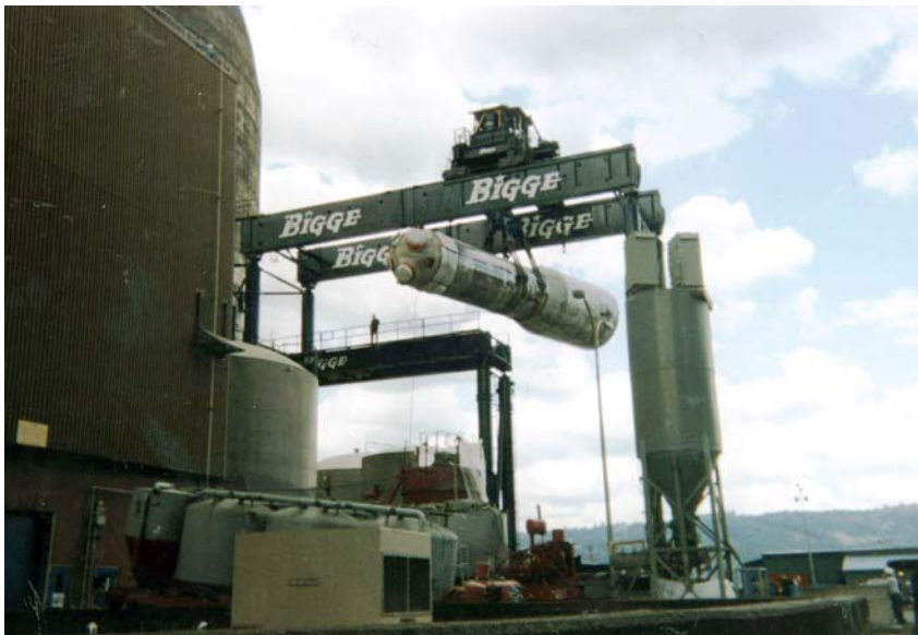
Figure 3 - A Steam Generator is Removed from a Reactor Building
