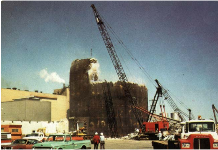
Figure 1 - Demolition of a Reactor Containment Building
