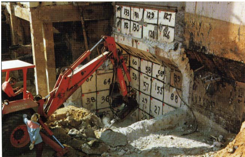
Figure 2 - Removal of Contamination on Nuclear Plant Wall
