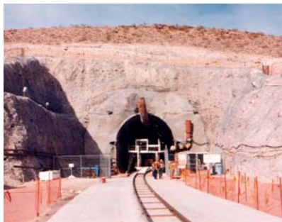
Entrance Tunnel at Yucca Mountain
