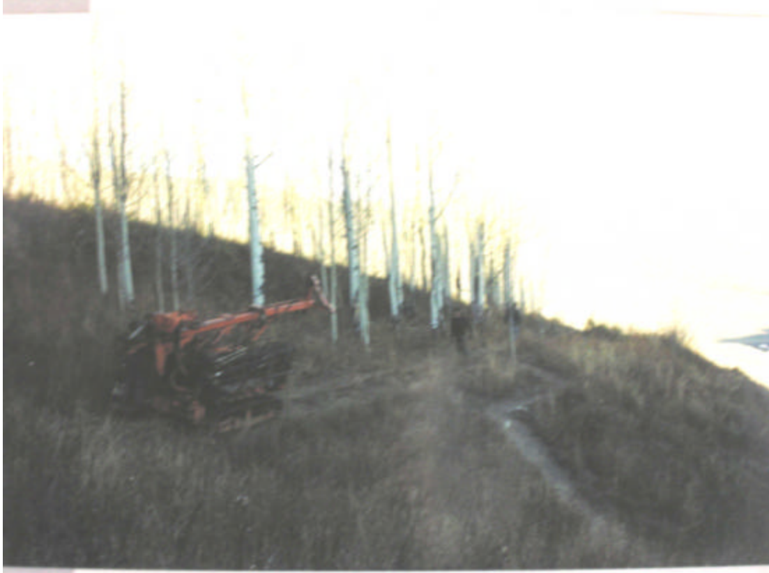
Fig. 6. Acker rig propelling itself at the top of the East Slide.
