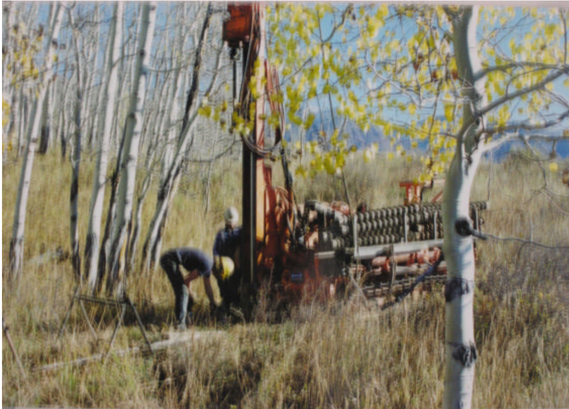
Fig. 8. Acker rig set up and drilling.
