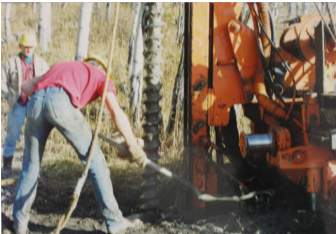
Fig. 9. Shoveling cuttings away from auger hole.
