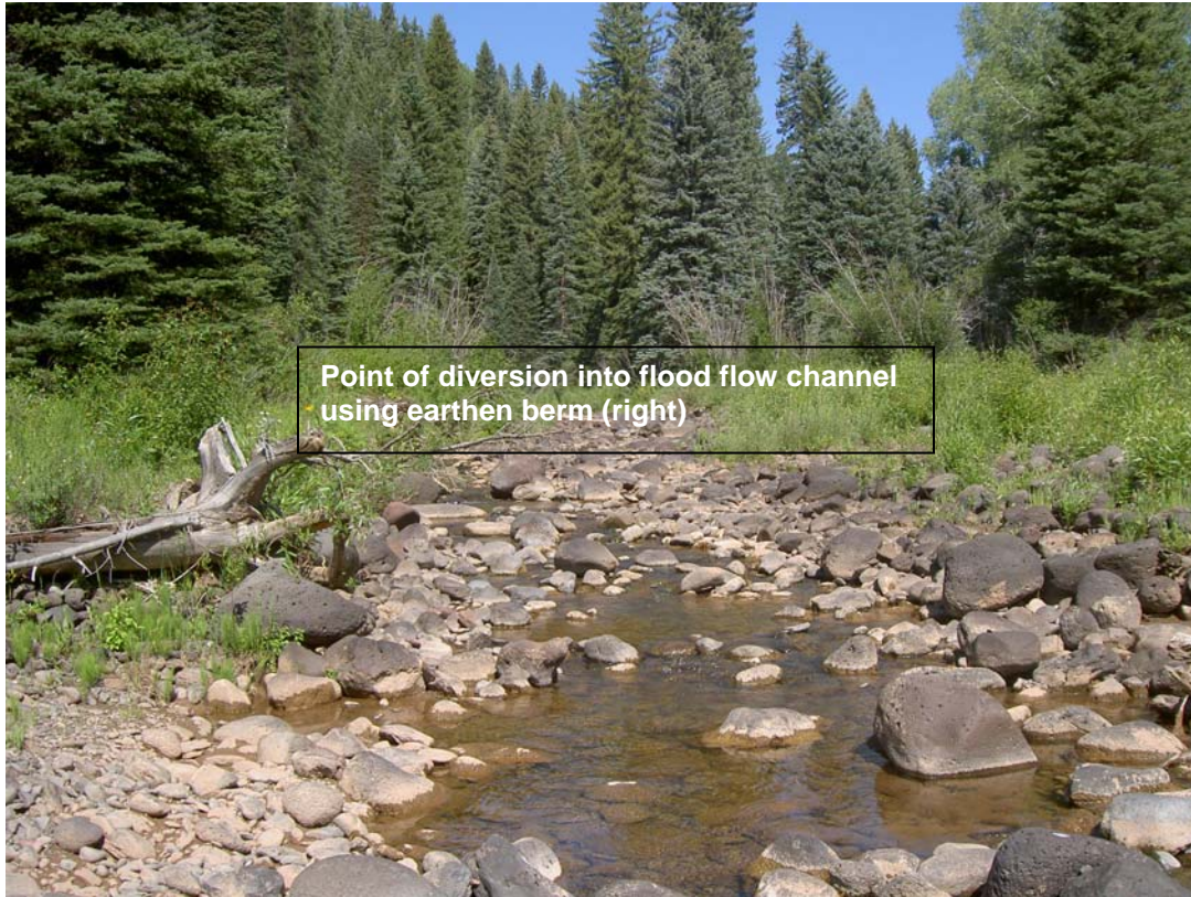
Figure 5 West Muddy Creek looking upstream from proposed crossing at point of diversion and earthen berm.
